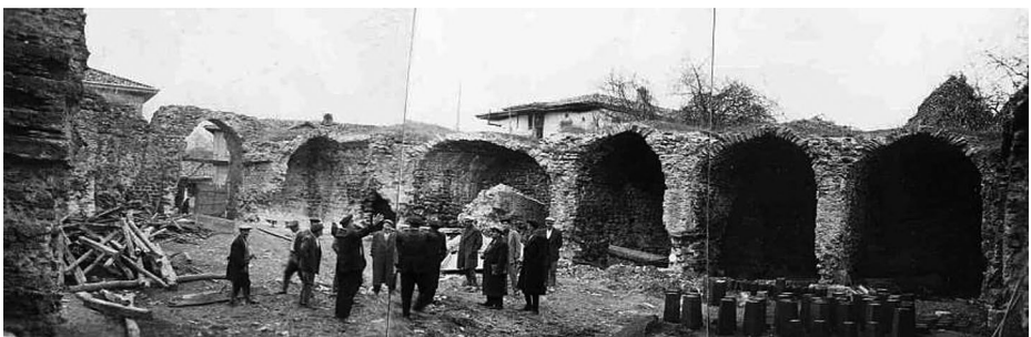
Photo 3 2nd period inn photograph-inn section (Conservation Report of Durak Han 2015)
