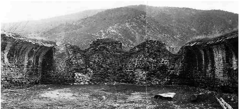
Photo 2 2nd period inn photograph-shelter section (Conservation Report of Durak Han 2015)
